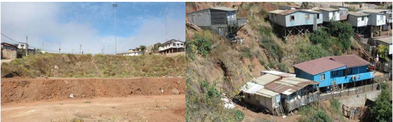
Figure 8: artificial terraces of the ravine heads (left), made to obtain construction areas (right).
