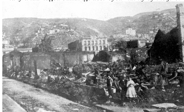
Figure 28. Damage at El Almendral, 1906 Valparaíso earthquake, showing backing the background the undamaged buildings and houses on the hills.
