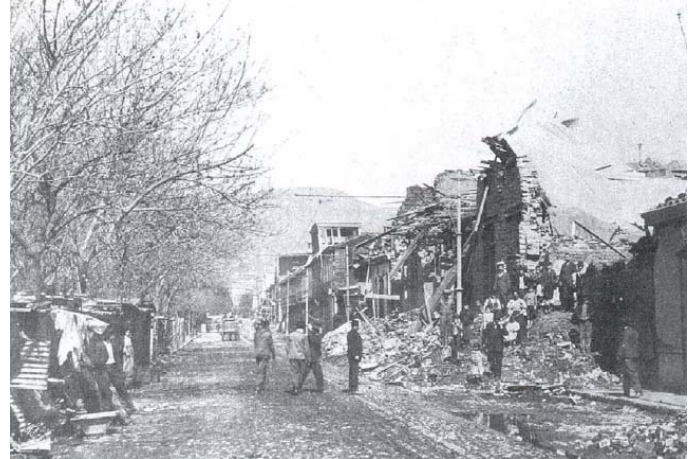
Figure 32. 1906 earthquake damage at Las Delicias Ave. (today Argentina Ave.) where the 1985 earthquake was recorded at El Almendral.
