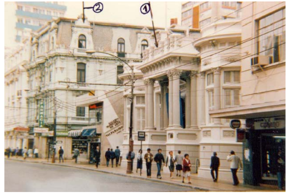
Figure 30b. Similar picture to Figure 13a taken after the 1985 earthquake again showing both undamaged buildings. Both buildings are Centennial since they survived both earthquakes.
