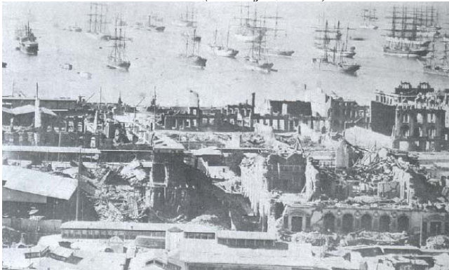
Figure 26. General view of the 1906 earthquake and following fire at El Almendral (picture from Bellavista Hill). The foreground shows the destroyed La Victoria theatre (La Victoria square) and, on the background, many undamaged buildings destroyed mainly by the fire.
