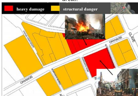
Figure 13. Explosion and fire in Calle Serrano.
