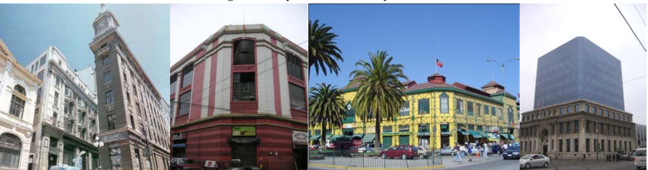
Figure 6. Valparaíso buildings in the flat area.
