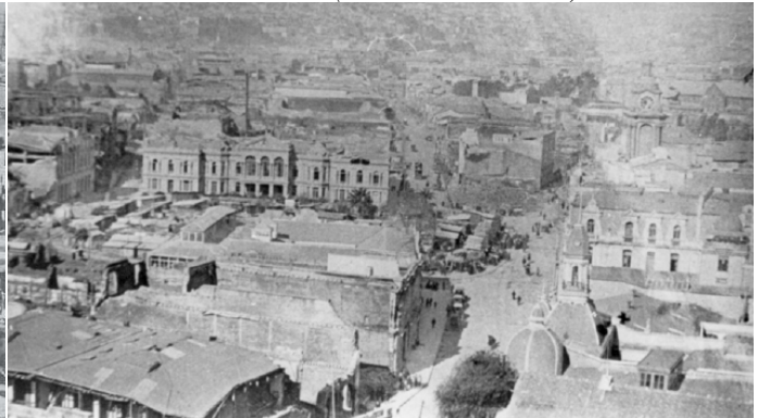
Figure 27. General view to the East of the damage due to the 1906 earthquake at El Almendral. At the centre of the picture, La Victoria square, showing the undamaged belfry of Espiritu Santo Church and the Huito building.
