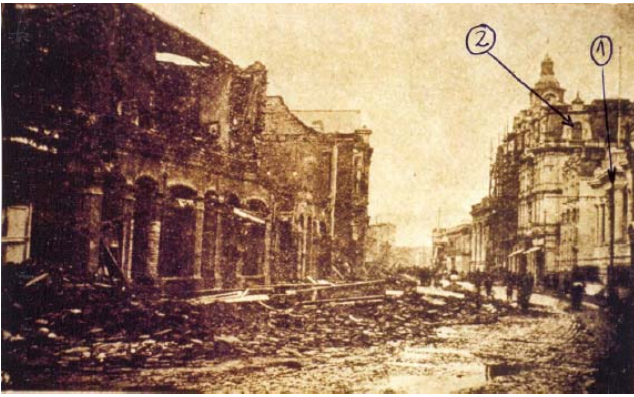
Figure 30a. Comparison between this picture taken after the 1906 earthquake of Condell Street near La Victoria Square, showing Lyon Palace (1) and 4-storey Huito building (2), undamaged, with picture of Figure 13b.
