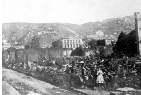
Figure 12. Damage at El Almendral, 1906 Valparaiso earthquake, showing backing the background the undamaged buildings and houses on the hills.
