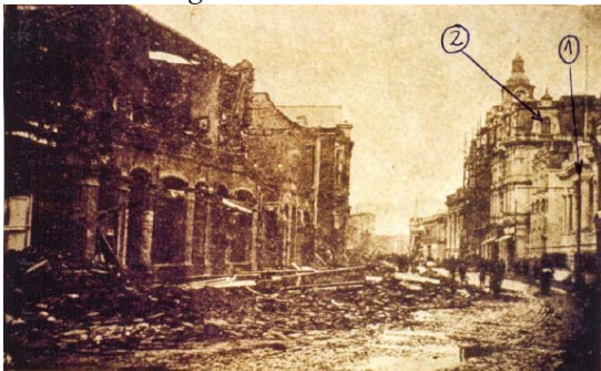
Figure 14a. Comparison between this picture taken after 1906 earthquake of Condell Street near La Victoria Square, showing Lyon Palace (1) and 4-storey Huito building (2), undamaged, with picture of Figure 13b.
