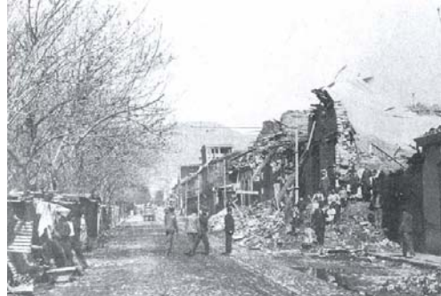
Figure 16. 1906 earthquake damage at Las Delicias Ave. (today Argentina Ave.) where the 1985 earthquake was recorded at El Almendral.
