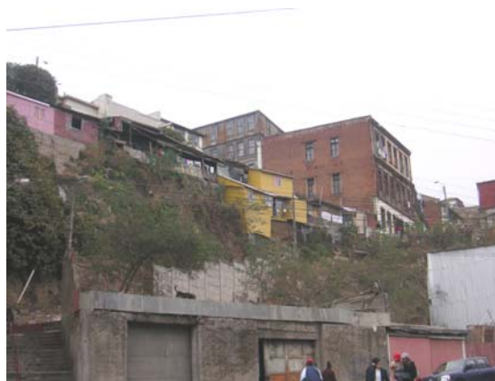
Figure 5: A “quebrada” with a potential risk of debris and mud flows.
