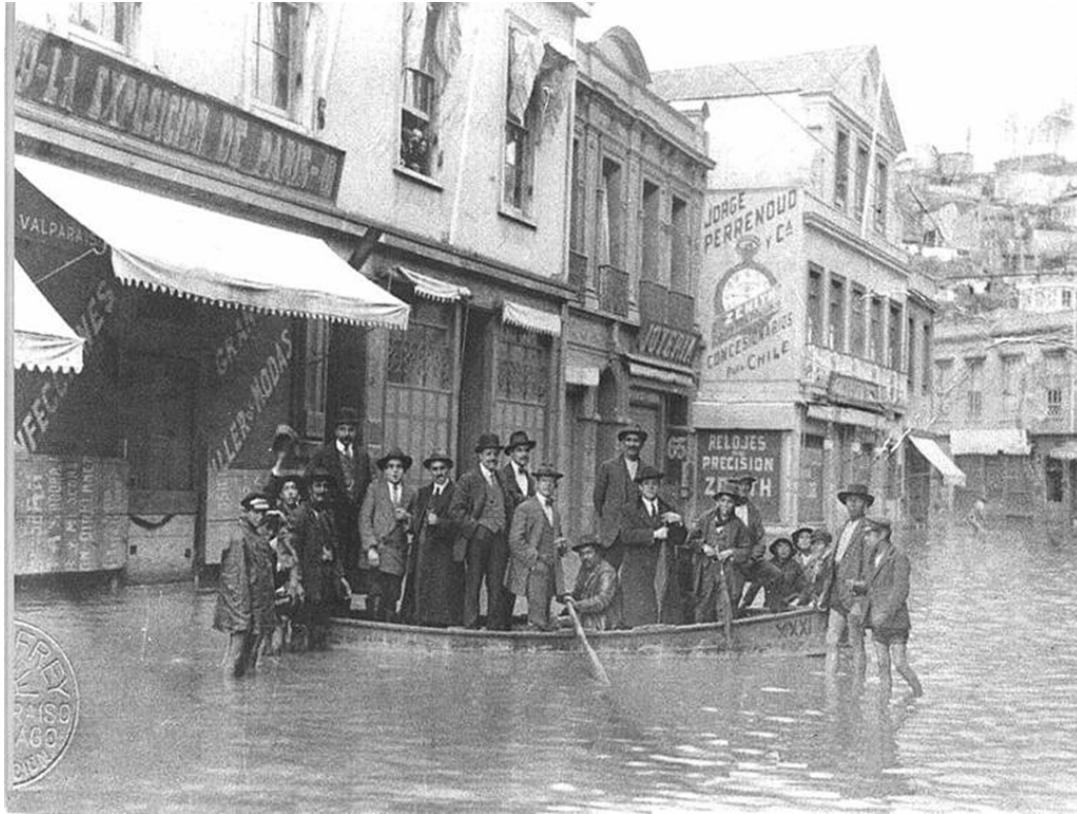
Figure 19. An old picture showing an inundation in Valparaíso.
