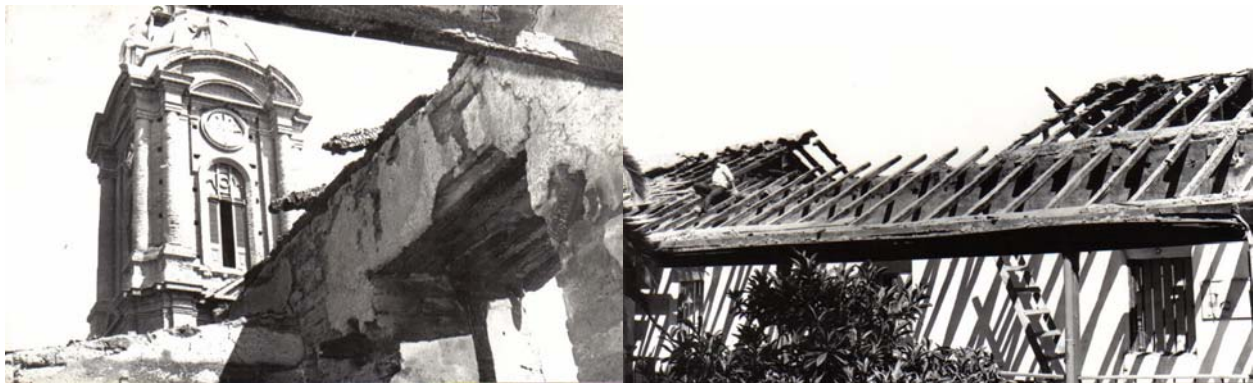
Figure 3: the San Francisco Church after the fire (1983).
