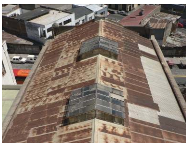
View of the roof covering
