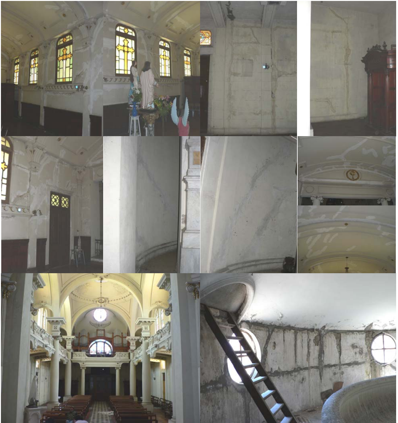
Figure 29: Some pictures of the interior of the Las Hermanas Chapel.
