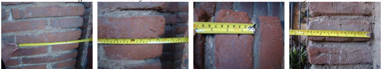
Figure 13: Masonry bricks of “San Francisco del Barón” Church.
