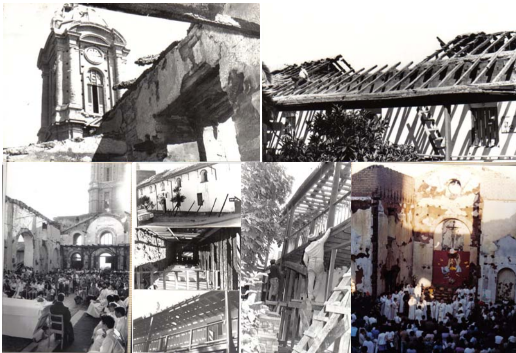
Figure 16: Fire damage in 1983 at San Francisco.
