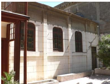
View of the West apse (chapel): some diagonal shear cracks are well visible in the lateral walls, between the openings
