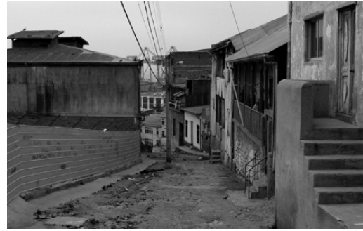
Figure 19: The existing condition of Calle Villagran.
